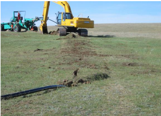
Plowing in pipeline installation technique. Photo Credit: S. Patey LeDrew
